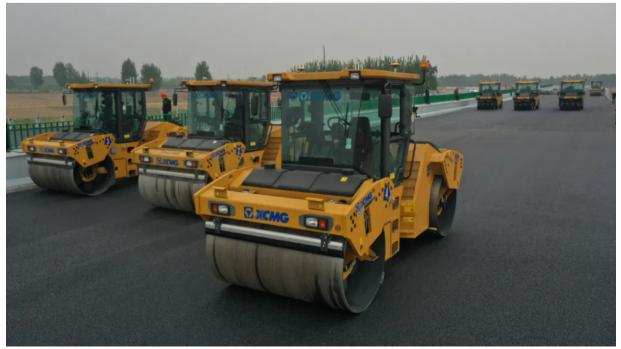
The machinery cluster adopts echelon operation, and is divided into a paving echelon and three rolling echelons of initial pressure, recompression and final pressure according to the operation process. The overall configuration of machinery and equipment is 2 pavers, 3 double-drum rollers (initial pressure, vibration pressure 3 times), 3 rubber-wheeled rollers (recompression, static pressure 8 times), 1 double-drum roller (final pressure), Vibration pressure 1 time).
