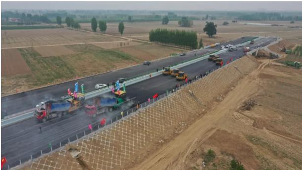
The test section of this paving is the right section of the main line K97+692.848~K98+095.5, 402 meters long, and designed to use 8 cm thick ARHM-20 asphalt mixture. The "unmanned cluster intelligent construction" technology saves costs and works efficiently. While achieving intelligent obstacle avoidance, it can track the rolling trajectory of the fleet and roller compaction data in real time, and the application of the drope cluster reduces the number of on-site personnel by two-
